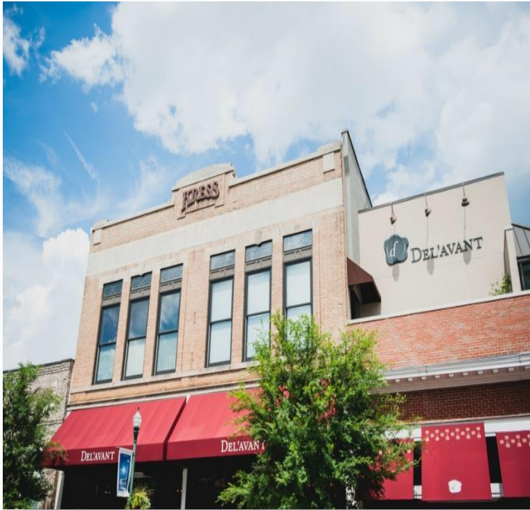
Figure 2: Historic Kress Building. Now Del'Avant Event Center
