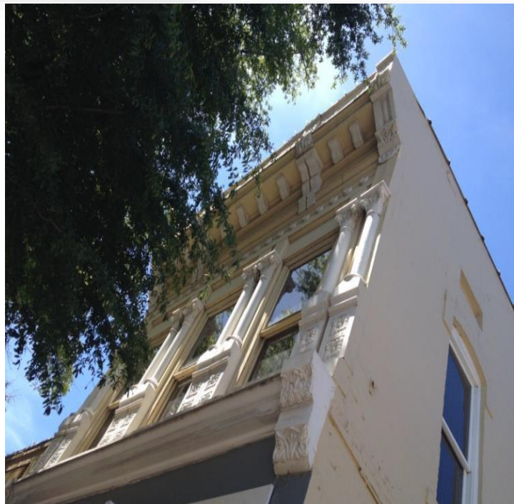
Figure 3: Downtown building containing historic metal facade.
