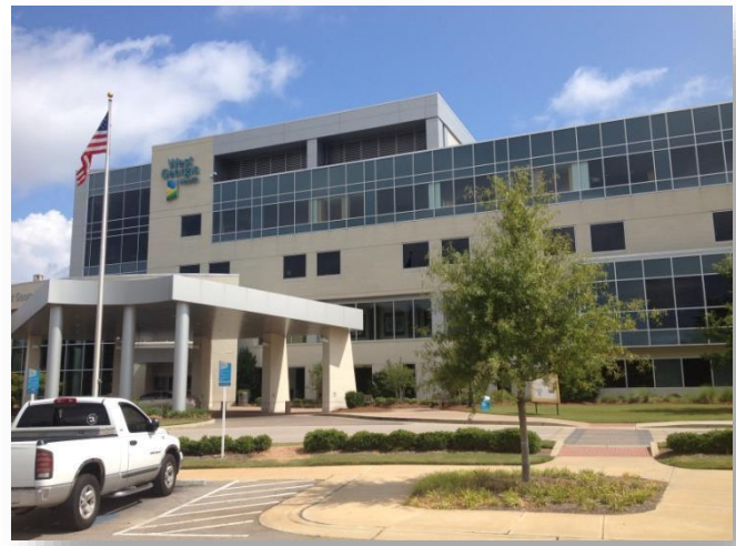
Figure 19: West Georgia Medical Center
