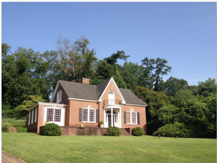
Figure 4: Traditional home in LaGrange
