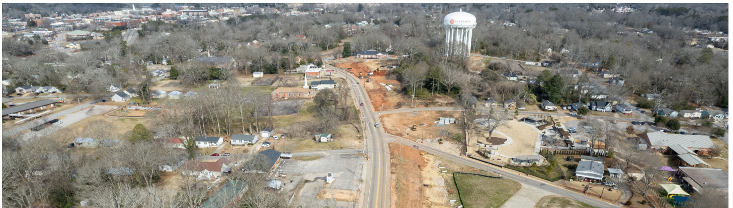
Hamilton Road Widening Project
